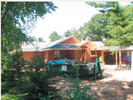
During construction phase
